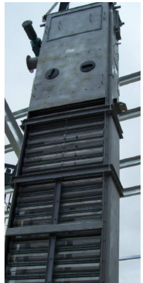
Installation of Eliminator Band Screen by crane.
