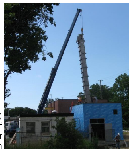
Pictured (right) Installation of Headworks Mahr Bar Screen
